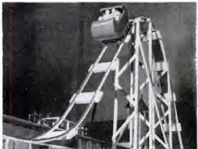
Roller coaster was 1953 addition. A chain pulls it to the top of tallest slide before its one-minute journey around island. A single \frac{1}{4} -horsepower motor beneath the platform powers every part of the display except the Wise Men on the wall above.
